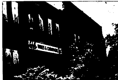
The old abandoned LaSalle winery on Grand River will soon become the home for several wholesale firms and a theme restaurant as its new owner finalized the real estate transaction last week and made plans for remodeling the 96-year-old structure. (Staff photo)
