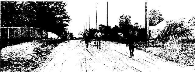
POWERS JUNIOR HIGH STUDENTS walk on Colfax Ave. on the way to school rather than on a gravel sidewalk built with Farmington School District funds. (Evert photo)
