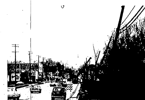
BEFORE -- Before workmen straightened them, the telephone poles along the front of the Valley View Apartments on Grand River tottered like falling 10 pins. (Evert photo)
