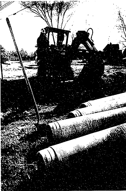
A Consumers Power worker reinforces gas lines along Greening Avenue, a preliminary step before water main construction. The asbestos water pipes in the foreground, a health worry for some residents, weren't installed as planned Monday. (Staff photo by Randy Bors)
