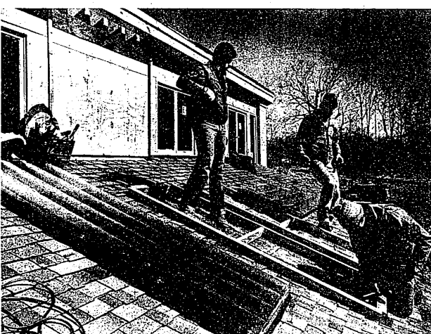
Installing solar panels for the home's hot water system are (from left) Joe Napolitano, Chris Endebrock and Glenn Mattox, of Star Pak Solar Systems in Novi. Above, an overview of the home which is half completed. (Staff photos by Randy Horst)
