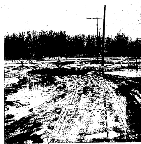
WATER, WINTER WONDERLAND—Residents on Canfield in eastern Farmington Township say lack of ditches along Canfield often floods their yards. Both Farmington Township and Oakland County disclaim responsibility for the ditches. A recent photo shows water from the ditches spilling onto the road. (Event photo)
