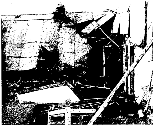
KINDERGARTEN ROOM. The kindergarten room of Eagle Elementary School at 29410 14 Mile Rd. was destroyed by fire Sunday night. The roof over the kindergarten area collapsed, leaving this open air view of the damaged room. Total damage to the school was estimated at $200,000. (Evert photo)
