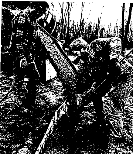
With mud to their knees, Dave James (left) and Dan Right keep the cement pouring.
