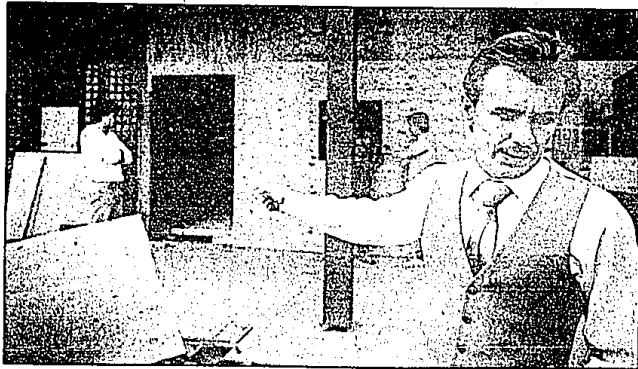
Al DuQuet points to the structural improvements being made to his Farmington jewelry store.
