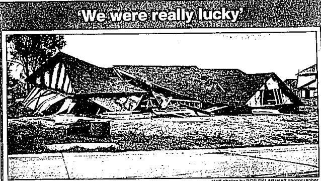
This house under construction on Derby Lane was lifted from its foundation, moved forward, then dropped.
