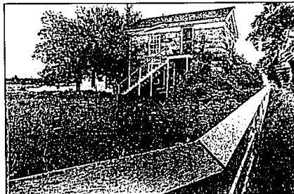
The historic Harger House has sat on a rise along Halsted, south of 11 Mile, for 150 years.
