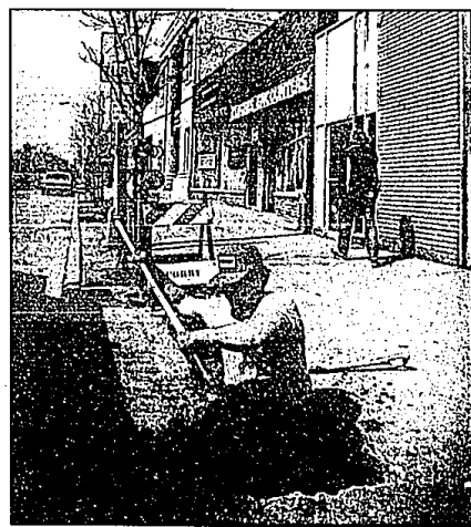
Scott Robinson of Corby Contracting digs a hole along Grand River where a new pedestrian lighting pole will be placed as part of the downtown Farmington streetscape project.
