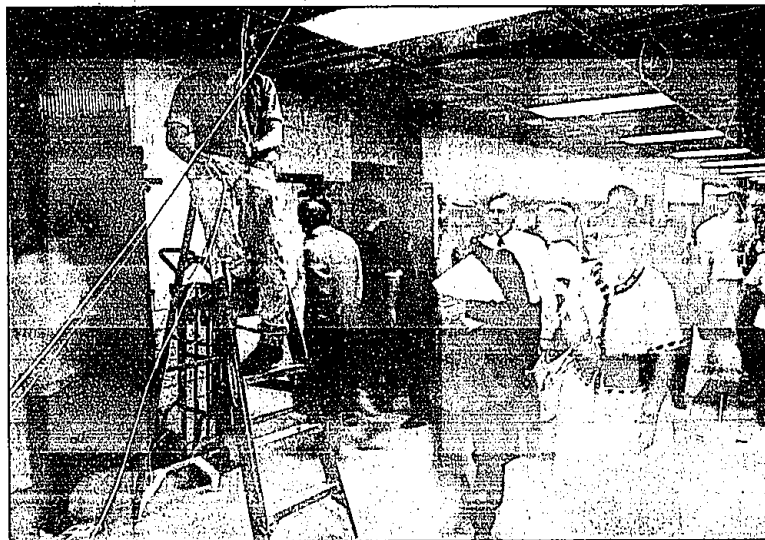
On tour: James Jackson of Datacom Solutions strings network cable in the halls of Farmington High School as the building tour group passes by. Work continues around the clock.
