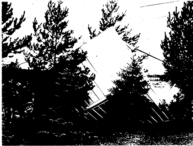
WIND DAMAGE -- Heavy winds left their mark on the Farmington landscape Friday afternoon with damage including a transported storage shed and a bent cross. The bent cross is attached to the roof of the Forest Hills United
