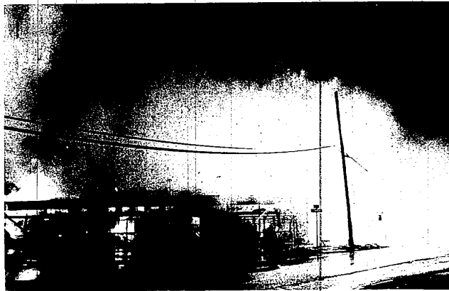
A WALL collapses with a burst of flame. Smoke blackened the sky and made it appear the sun had set early. (Photo by Ralph Evert)
