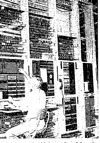
FINAL TESTS are now being made on all equipment in the new Bell Telephone Building at Grand River and Powers Road in preparation for the change over to the dial system in Farmington this Sunday, August 21. Huge test-beds will be used to determine if any and all troubles which may develop in connection with the new direct dialing system in Farmington, both during the change over and after the dialing system has been in operation.
