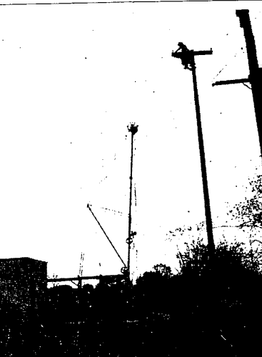
WELL DRILLING operations were started the latter part of last week at a new site on the Middlebelt Elementary School property in hopes of finding a more suitable supply of water. Utility wires on Ten Mile Road had to be raised before the driller's rig could be set up and placed in operation. The drilling of the well was deemed necessary following the disclosure that large quantities of sand were being brought up from the present well along with the water, causing damage to the pump and other well equipment.
