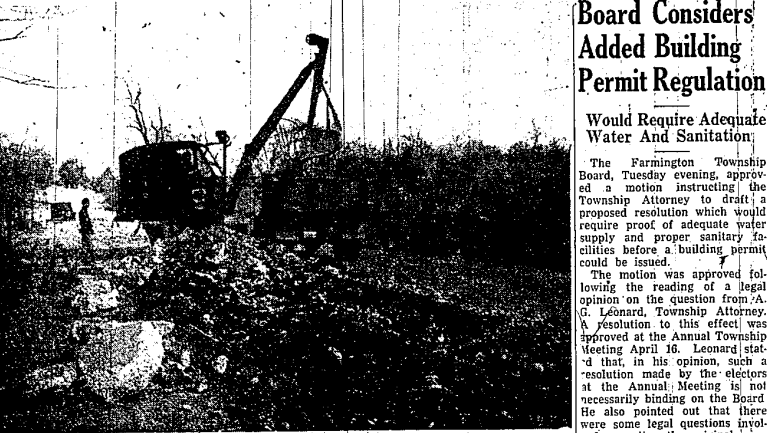
ROAD PATCHING work is well under way on a 1.36 mile stretch of Ten Mile Road extending from Power Road in Farmington to Telegraph Road in Southfield. Concrete patching of the entire length was the first phase of an overall resurfacing program is scheduled for completion on or before July 15. Work will be started soon afterward on the complete resurfacing of the main east-west highway with bituminous concrete, the Oakland County Road Commission disclosed. The above picture, taken last week just east of Woodhull Subdivision, shows a shovel engaged in clearing broken concrete from a portion of the road, to be filled with new concrete base.
