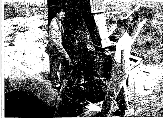
FINAL TESTS on the newly constructed city sewer interceptor were completed early last week in preparation of the opening of the system on Thursday. Earl Scherffus, City Manager (left) and Norman Knapp, newly appointed superintendent of the water and sewer department, examine the grid removed unit shortly after the system was placed in full operation. The grid removal unit along with the storm water treatment plant are located on the north side of Nine Mile Road east of Brookdale.
