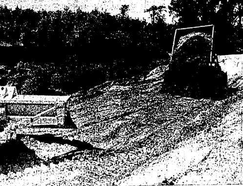
A LOT OF DIRT has been dumped in the past week and a half in an effort to bring that portion of Hatsted Road north of Grand River which was in a week ago Sunday back up to grade and make it passable.
