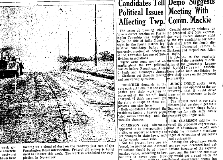
DUST WAS REALLY flying last week as work got underway on the preparing of the concrete underpass near the Orchard Lake Road westward to Haggerty Road. Heavy leveling equipment is shown here turning up a cloud of dust on the roadway just east of the Farmington Road intersection. Federal aid money is being used to finance this work. The work is scheduled for completion in November.
