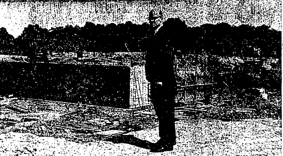
THE NEW BOTSFORD GENERAL Hospital is being built on land to the east of Oxford just south of Independence street, behind Botsford Inn. The four-story structure is not expected to be ready for use before 1965.
