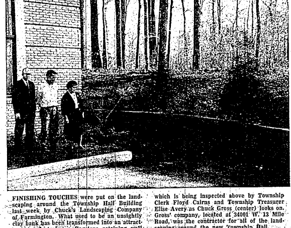
FINISHING TOUCHES were put on the landscaping around the new Township Hall by Chuck's Landscaping Company of Farmington. What used to be an unsightly clay bank has been transformed into an attractive area featuring a flagstone retaining wall
