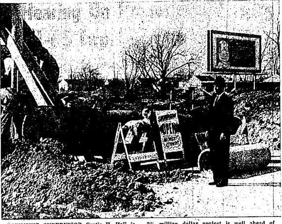
TOWNSHIP SUPERVISOR CURTIS H. HALL is pictured above inspecting the installation of water transmission lines at Middlebelt and Nine Mile roads where construction on the
