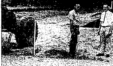
THE MAGIC SQUARE at the Flanders Eiche Elementary School which has raised much concern over the past several months at City Council and the school board is now under construction and expected to be ready for use next month. Flanders School principal Frank Delewski (left) is pictured above inspecting the construction with Farmington City DPW Superintendent Floyd Sallow. The magic square will provide a multi-purpose recreational use to benefit youngsters.
