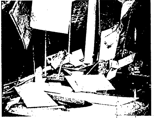
THE PIT STOP at 23830 Farmington Rd. in the City of Farmington lost its ceiling last week. This was the scene the next day. Investigators were examining the incident to discover just what had caused the fire.
