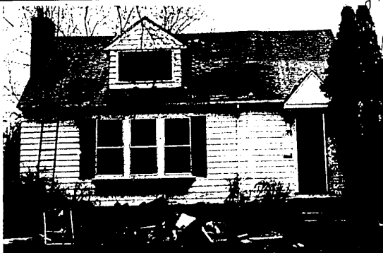
THE FIRE WHICH RAVAGED the Fred Hamlin home of Brookdale last Wednesday afternoon was contained by firemen to the upstairs portions of the house where the blaze started. Firemen battled the flames for half an hour before bringing the fire under control. The gaping hole in the roof and the pile of charred furnishings in the front yard lend mute testimony to the destructive force of the fire.
