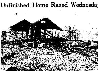
Only the garage and the foundation walls remain of the unfinished Charles A. Bronson home on Valley Drive in Wood Crest Farms subdivision after fire last Wednesday night razed most of the $15,000 house.
