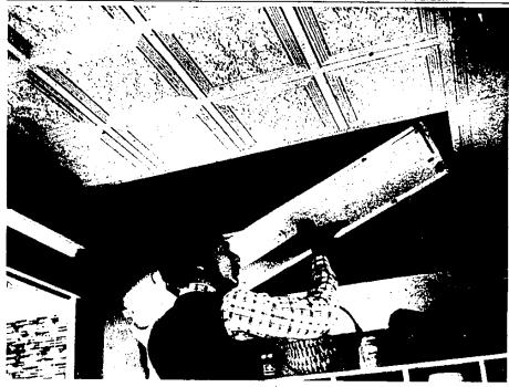
Suspended ceilings, like the one pictured, provide flexible systems for arranging and rearranging light fixtures. Recessed fluorescent fixtures, which supply efficient and low-cost Illumination, simply snap onto the grid above the level of the new ceiling.
