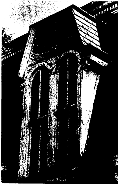
Although the ravages of time and weather are almost invisible from the ground, the temple's dormer windows need a fresh coat of paint and new panes. The slate roof eventually will be repaired also.
