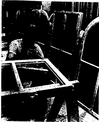
George McFarquhar carefully trims a new dormer window with white paint. There are 23 separate operations involved in restoring one of the old panes, according to McFarquhar.
