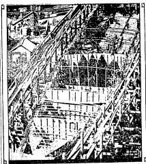
This view shows the U. S. destroyer Ward, under construction at Mare Jaland navy yard, California, 24 hours after the keel was laid. As mu structural work as possible was prepared in advance; bulkheads, sections the keel, deckhouses and bridge structure were rivered up rendy for assembling place on the ways. The Ward was launched 17½ days from the date laying of her keel. This is a new world's shipbuilding record.
