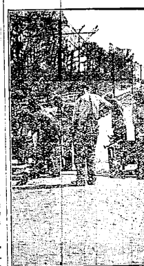
Vitrified Brick for Paving Country Roads—Filling the Joints, First Coat.
