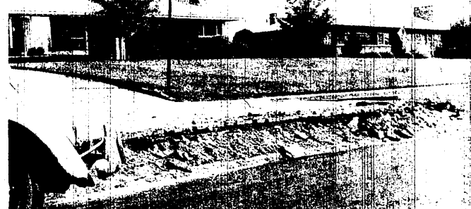
NO DRIVEWAYS — That's the problem in the Alta Loma Subdivision as the roads are re-surfaced. The work, which has been running behind schedule, is expected to be completed in the next week. The city will grade the driveways down to the street level, but the residents
