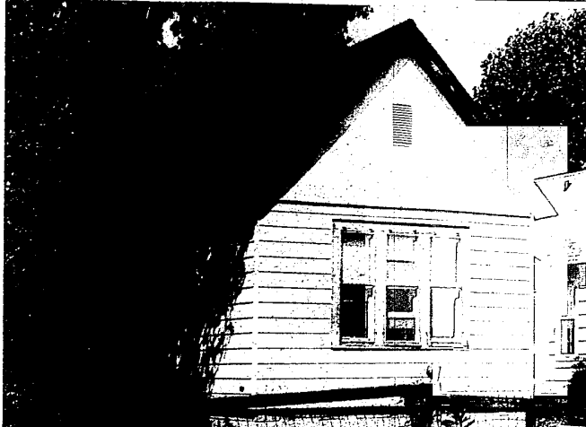
CLEANUP PROGRESS -- Part of Ralph Bell's work involves advising and working with residents who want to help themselves. This home is the result of Bell's work with a homeowner who dressed up his residence with aluminum siding. (Evert photo)
