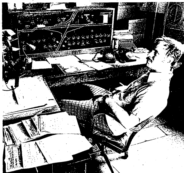
Joe Crawford relaxes before the switchboard at the Plymouth yard. The board keeps exact track of where each train is, preventing them from running into one another "even if the engineers tried." (Staff photo.)
