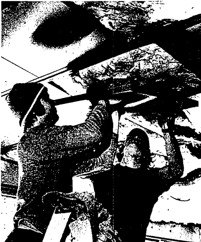
Sol-Ar-Tile panels weigh 43 pounds each. They can release approximately 465 BTUs of heat over a 10-degree cooling range. As these workers show, they are easily installed.
