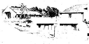
An underground house has earth and grass on three sides and is open to the sun on the fourth side, (Copyside) and is open to the sun on the fourth side, (Copyside)  $\frac{1}{2}$
