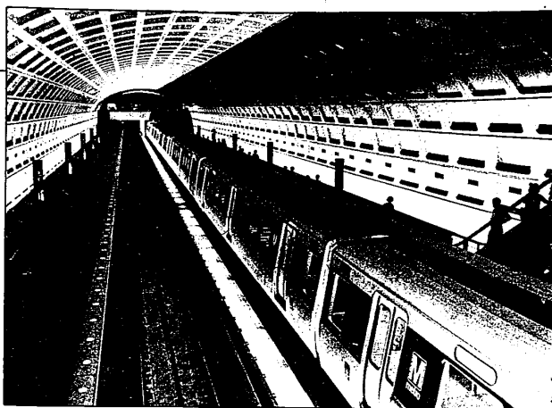
Metrorail stations feature attractive and functional barrel vaulting which helps deaden sounds. Compared to subways in New York and Chicago, Washington's system is cathedral quiet. Floors, stairs,
