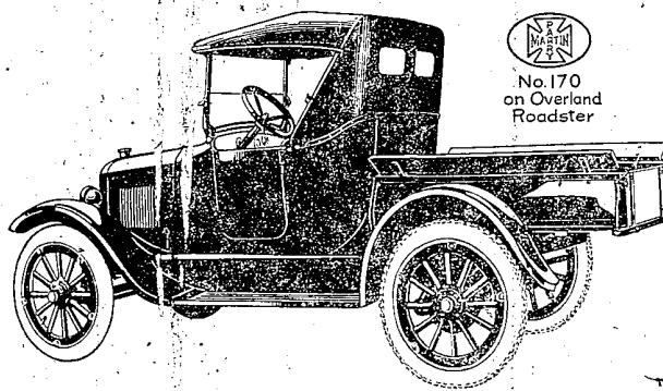
In the Overland Roadster you are getting practically two cars for the one price. The turtle-back is quickly removed to permit the substitution of a box panel, or a light express flare-board body. These slip-on bodies fill a big need in the day's work of the merchant and the salesman.
