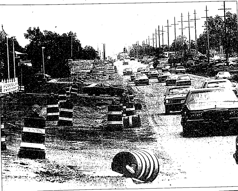
LEFT: Temporary roads will be constructed on Orchard Lake Road south of Maple in West Bloomfield so traffic may continue while the road is widened. ABOVE: A truck drops a load of dirt to prepare the temporary road. BELOW: It's the "sign" of the times on Orchard Lake Road where reconstruction to widen the road continues until December.
