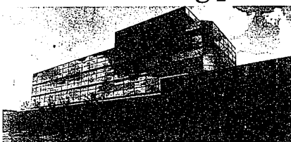
Panels from the glass facade of Jan and Don O'Dowd Hall at Oakland University have been popping out of place. All 494 panes will be replaced by the manufacturer at no cost to the school or state. (Photos by David Frank)
