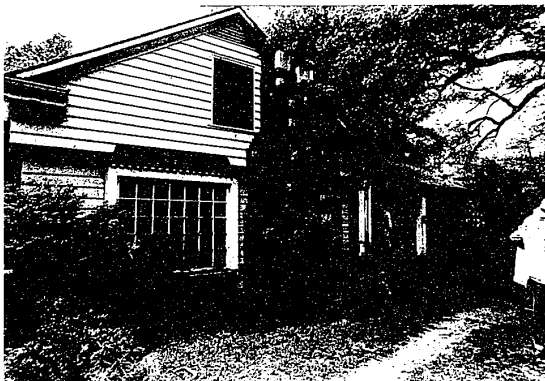
The Bruner home in West Bloomfield stands on a bluff overlooking Pleasant Lake. Erwin Bruner built the home 40 years ago.
