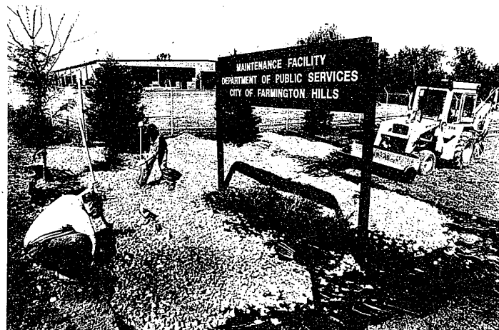
Maintenance never stops for members of the Department of Public Services (DPS) crew. In the foreground Tom Young, and in back Eric Man, follow a design they made to revamp a plot with wood chips on the DPS grounds.
