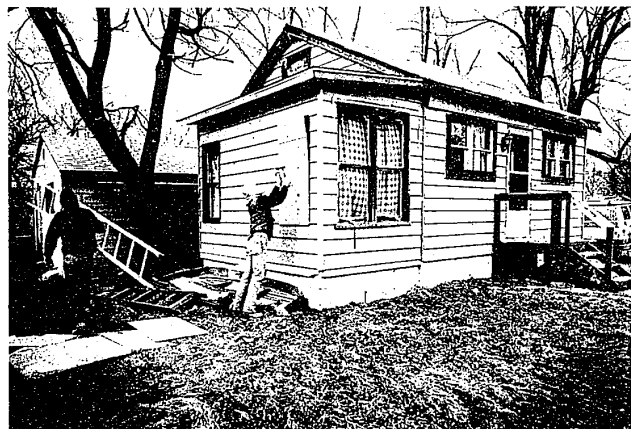
Boarding up an abandoned home on Ontaga at Emmett are Dennis Maier (with ladder) and Bob Lewis. Neighbors say these vacant homes are hav-
