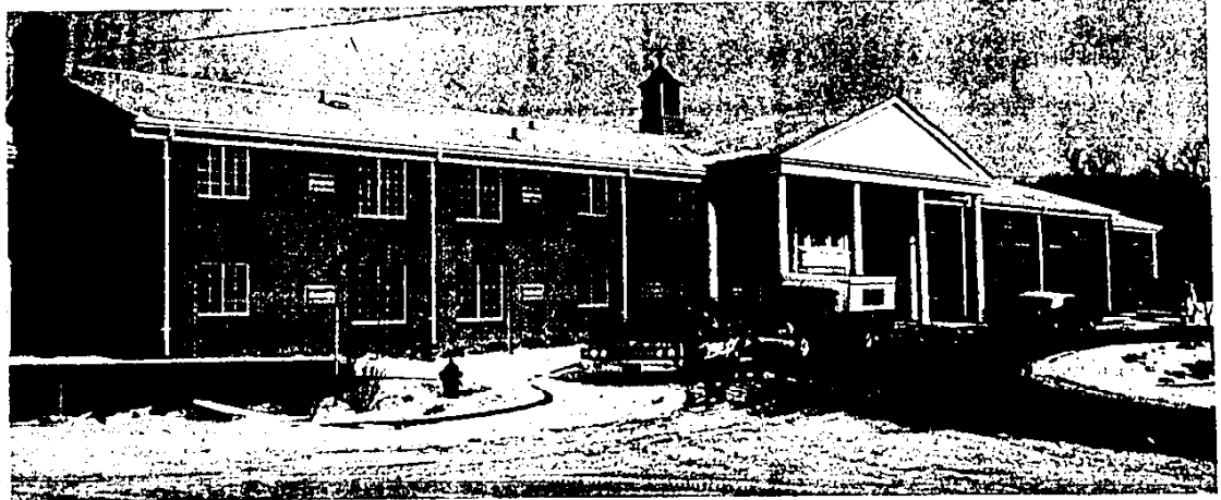
TONQUISH CREEK MANOR is the name given to this Plymouth senior citizens housing project of 60 apartments which will be open to residency this spring. Representing expenditure of $1 million in construction costs, the manor
