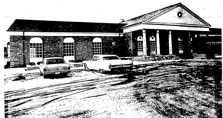
NATIONAL BANK OF DETROIT, which operates two branch offices in Plymouth, will open a third facility (this spring) nearing completion. The colonial styled structure is located at Sheldon and N. Territorial Roads. (Observer photo).
