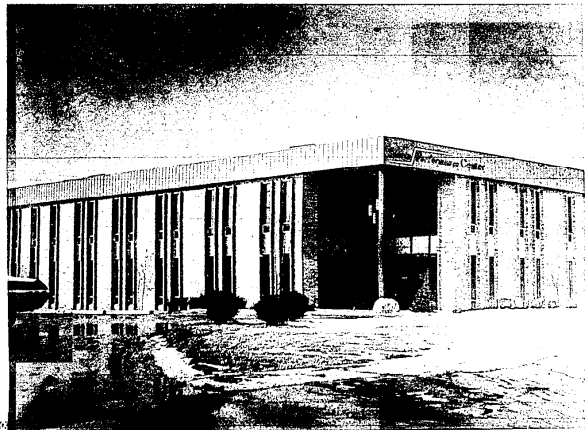
GOING UP and rapidly nearing completion is the new K-Mart store near the Wandafield Shopping Center in Livonia. The huge structure (above) is scheduled to open in the near future and will provide another K-Mart outlet in the communities covered by the Observer Newspapers. (Left) A new addition to the Livonia industrial community is the Sports Performance Center. It is located in one of the city's three industrial parks.
