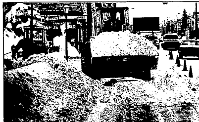
Robert Hope mans the front-end loader to clear the sides of the street while Kirk Schade (left) works on the sidewalk.
