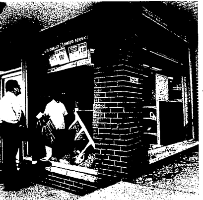
Damage to the building's exterior is inspected by Jay D. Harrison, building inspector for the city of Farmington while Harry Watson, store owner, surveys the damage done inside the store.
