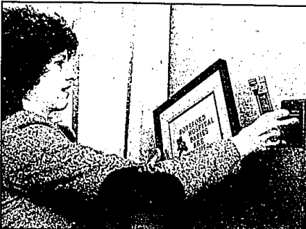
Oxygen outlets are hidden behind pictures on the wall. There are two on each side of the bed, one for the mother and one for the baby.
