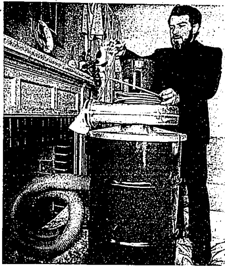
Gilreath uses a large vacuum cleaner to insure that soot will not enter the house.
